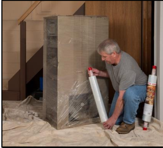
Wrap the unit completely
